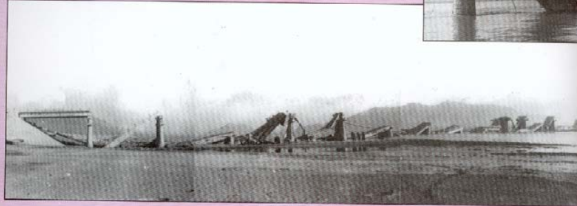
唐山地震中被震毀的灤河公路橋 The highway bridge over Luan River deformed in Tangshan earthquake.
