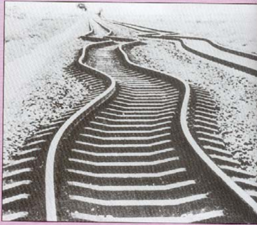
唐山地震中被震毀的鐵道線 Railway tracks deformed in Tangshan earthquake.
