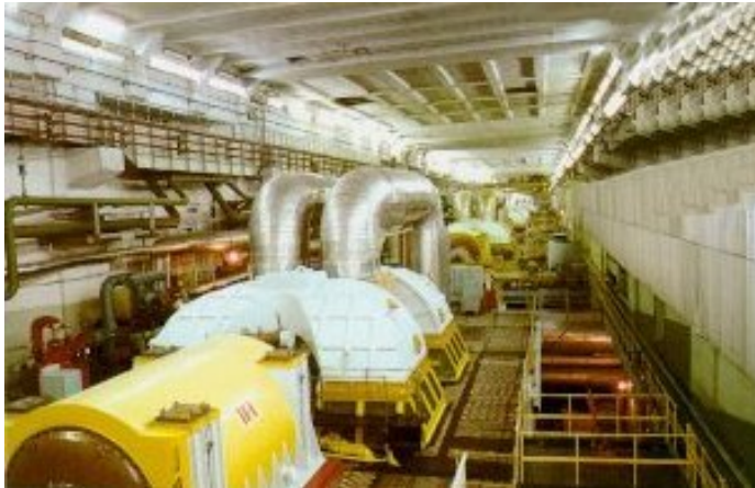
Turbines and generators hall
