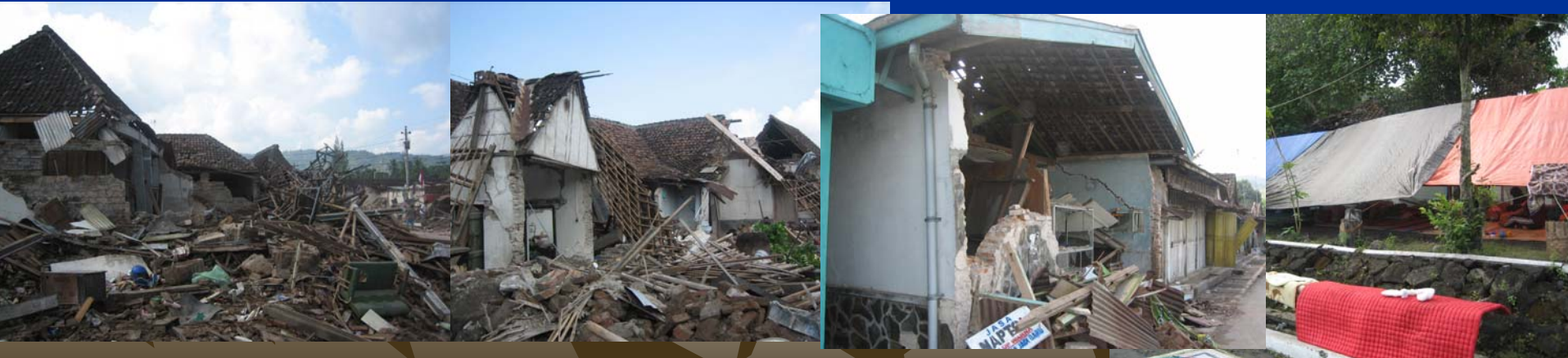
Pictures of damaged houses and disaster distribution in Imogiri
